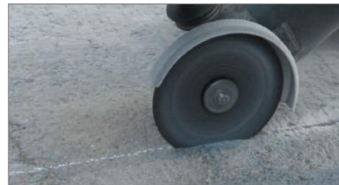
Picture 3 – Cutting the edges of the repair area
