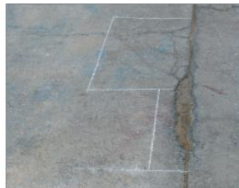
Picture 2 – Determination of the borders of the repair area
