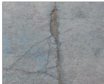
Picture 1 – Determination of the repair area
