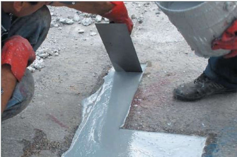
Picture 8 – Concrete floor repaired with StenCare®
