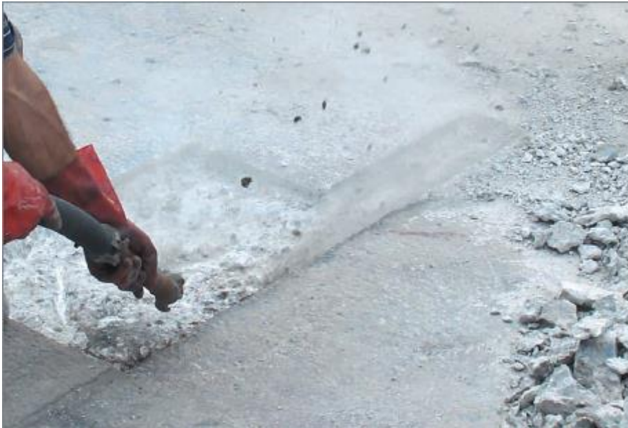
Picture 6 – Cleaning of the repair area
