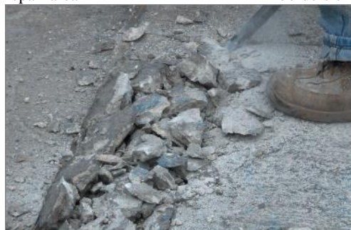
Picture 4 – Clearing out the repair area
