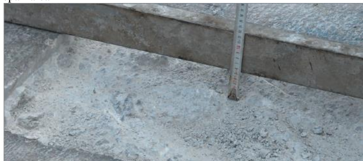
Picture 5 – Adjusting the depth of the repair area
